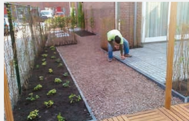
TTE®: with gravel backfilling, wooden superstructure and TTE® paving stones (NL)
